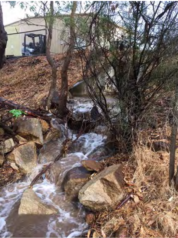
Above: Water cascading over the rocks below the outlet and spillway.
